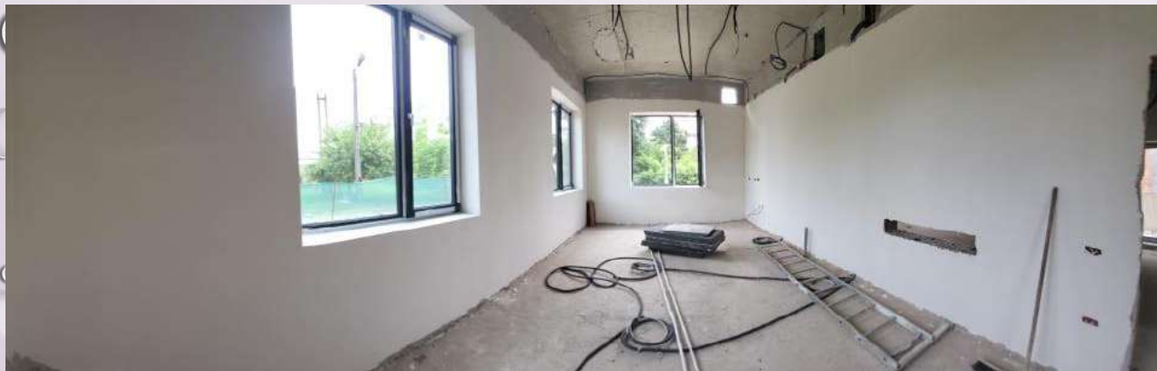
C20 and C21 buildings - the final stage of rehabilitation
